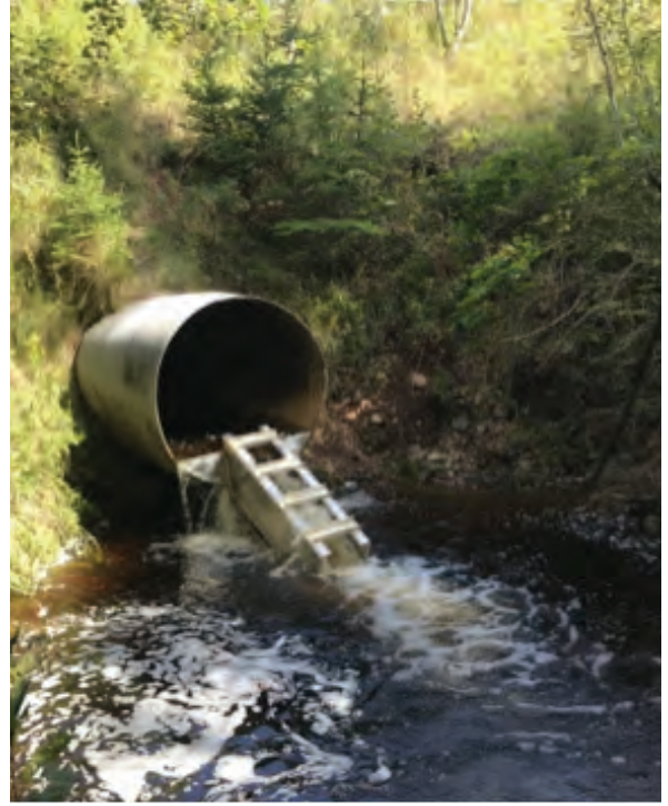
Images taken after construction (Upstream/Downstream) and Installation of the Alaskan Steeppass Denil System on the Folly River, Lower Debert, Nova Scotia. Photo Credits: Blake McNeely
