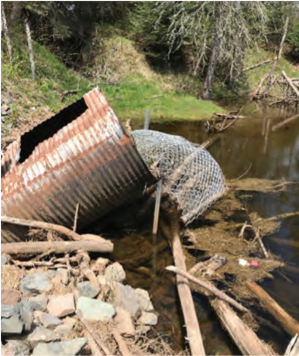
Images Taken Before Construction (Upstream/Downstream) of the Installation of the Alaskan Steeppass at the Severely Damaged Culvert located on the Folly River, Lower Debert, Nova Scotia. Photo Credits: Blake McNeely
