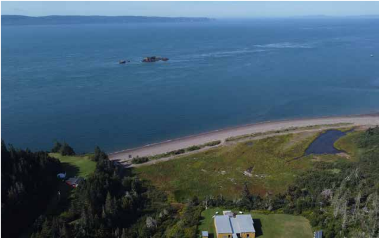
Figure 2 Aerial View of Fundy Ocean Research Center for Energy (FORCE) in Parrsboro, NS
