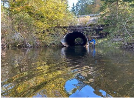
Figure 4: Outflow After Restoration Activities
