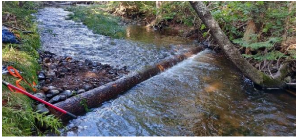
Figure 8: Downstream of Digger log Installed on Cook Brook, Portapique, NS
