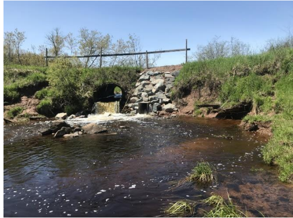
Figure 1: Downstream of Newly Installed Denil
