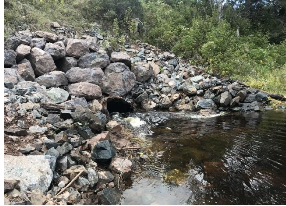
Figure 7: Upstream of the Folly River Culvert
