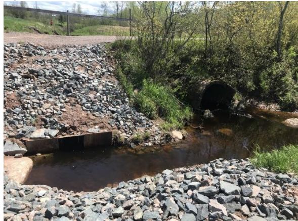
Figure 2: Upstream of Newly Installed Denil
