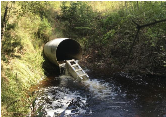
Figure 6: Downstream of the newly installed chute system
