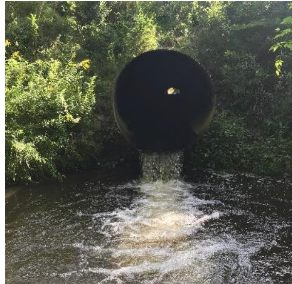
Figure 5: Downstream of the Folly River culvert
