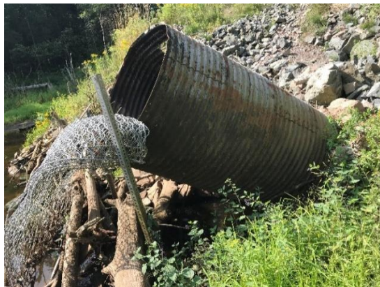
Figure 4: Upstream end of Folly River Culvert
