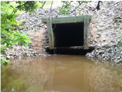
A wooden culvert with low water levels fragments the watercourse
