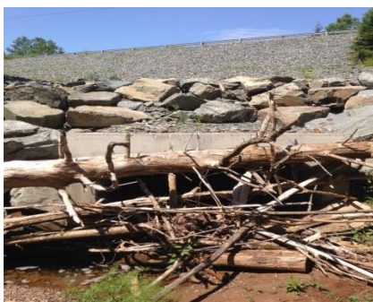
Debris blocking concrete culvert and fish passage
